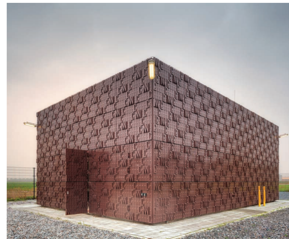
Afb. 1.4 Gasontvangstation Dinteloord, 2012; Architect: Studio Marco Vermeulen Foto: Ronald Tilleman
